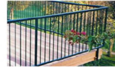
1. METAL VERTICAL RAILING
